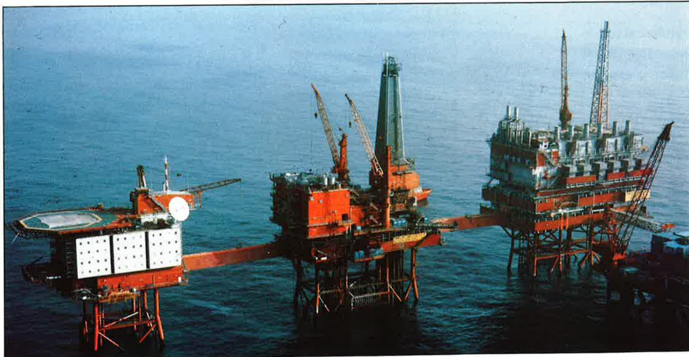
The Valhall Field has produced 130 mill. barrels of oil since it came on stream in 1982.
